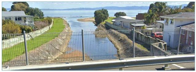
Figure 30: Tararu Creek looking downstream, note the proximity of dwellings to the top of bank
