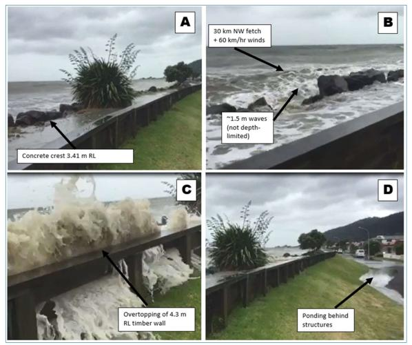
Figure 6: Waves overtopping Moanataiari defences on the 5 January 2018 (Note levels indicted are m MVD53)
