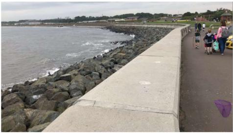
Figure 9: Example of concrete wall flood defence
