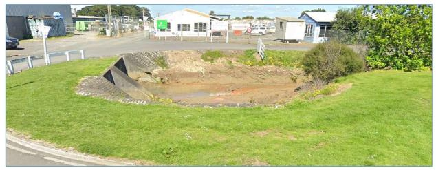
Figure 37: Head of exposed drain - limited space and erosion prone with the culverts and drains requiring one-way flow valves
