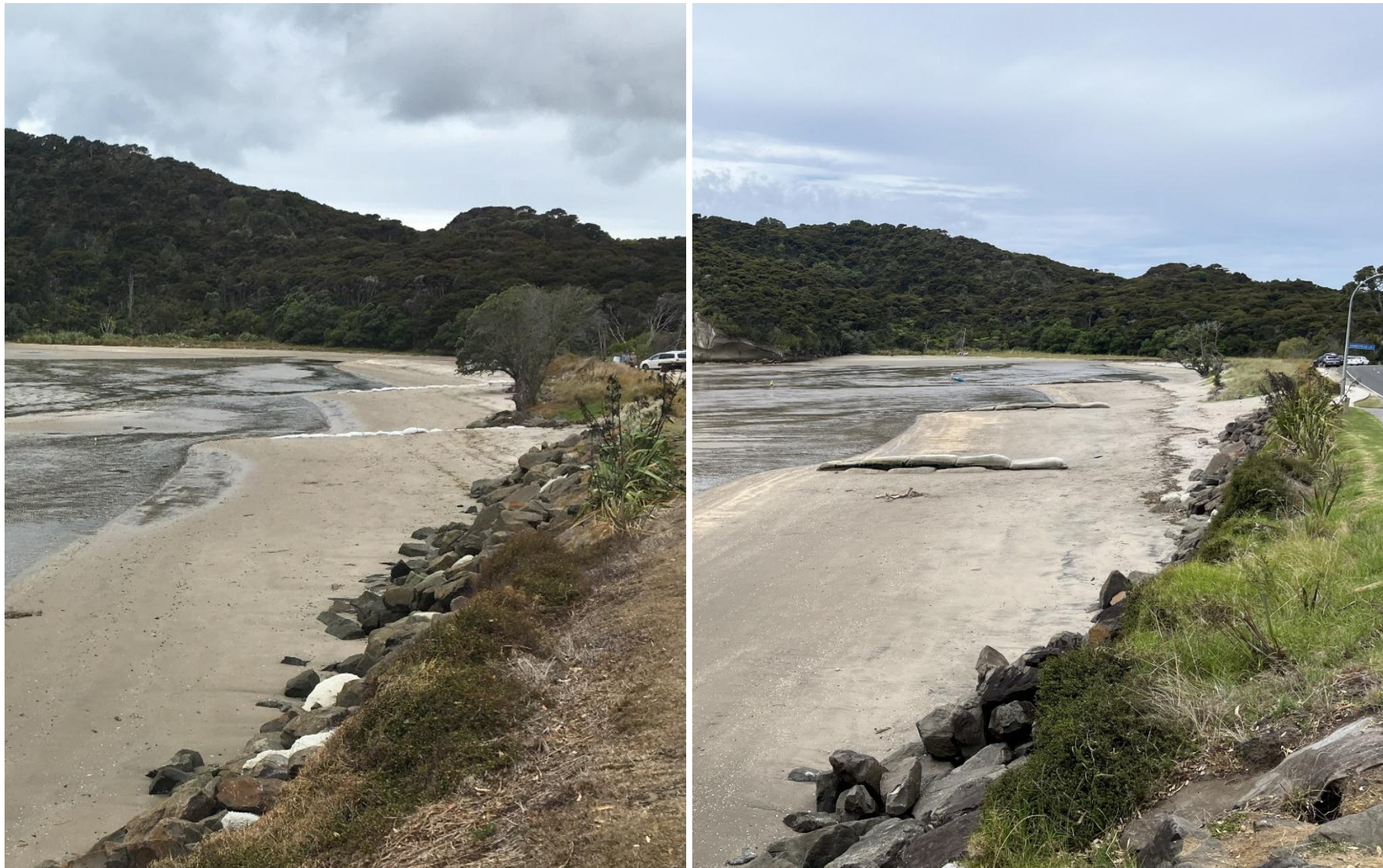
Figure 3: Flaxmill Bay in March 2020 (left), showing unconsented groyne structures constructed by a local resident and in February 2025 showing the three consented geotextile groyne structures (right).
