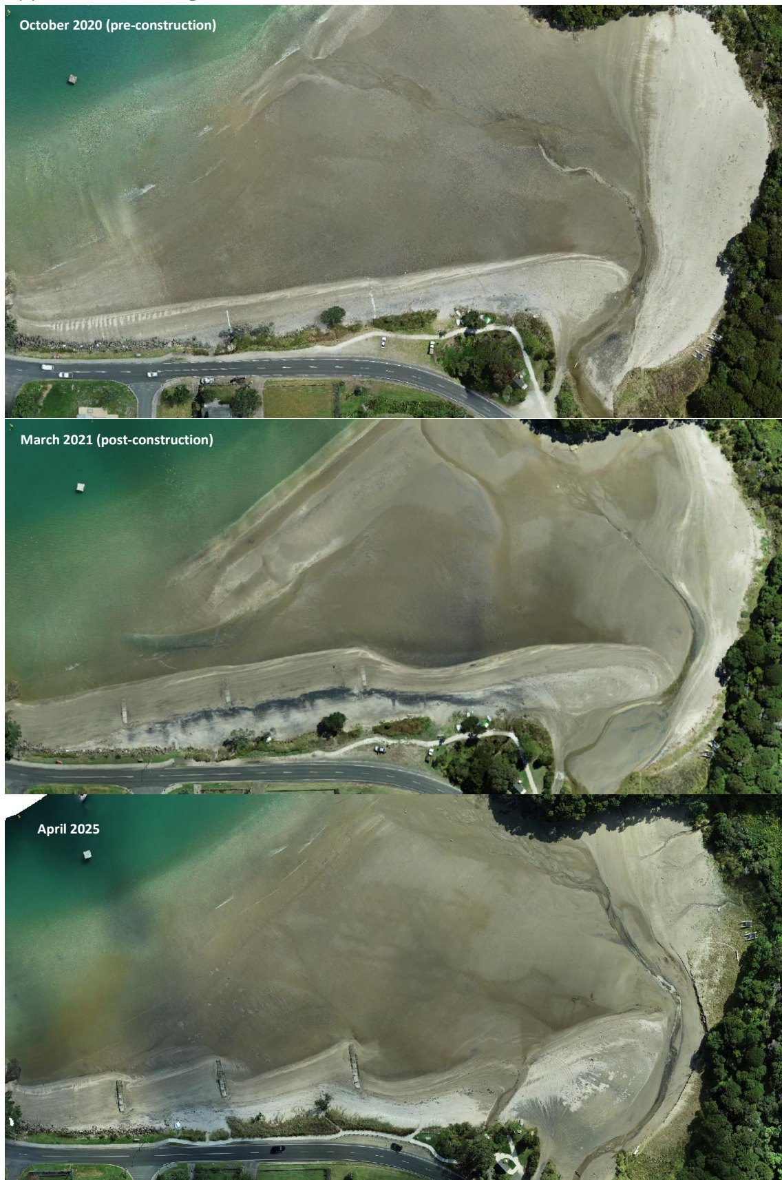
Figure 12: Changes in sediment distribution and shoreline position from pre-construction (top – October 2020), post construction (middle – March 2021) and most recent (bottom – April 2025).
