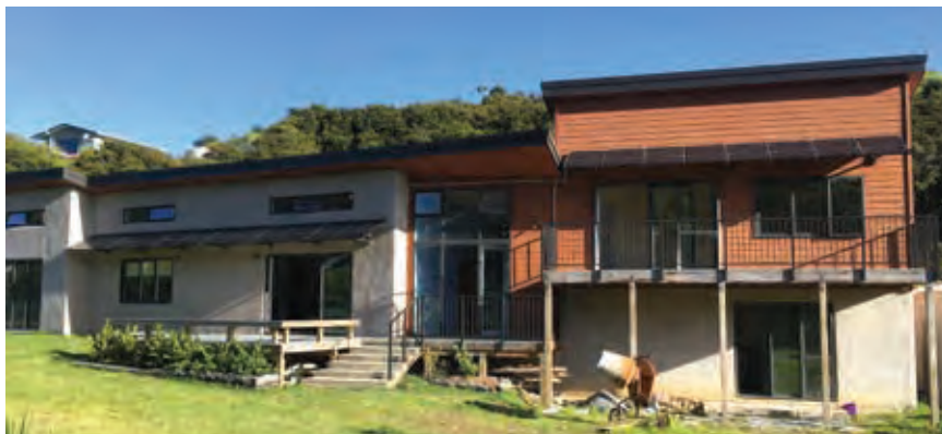
▲ Glazing on the north side soaks up sun in winter to heat the home.
