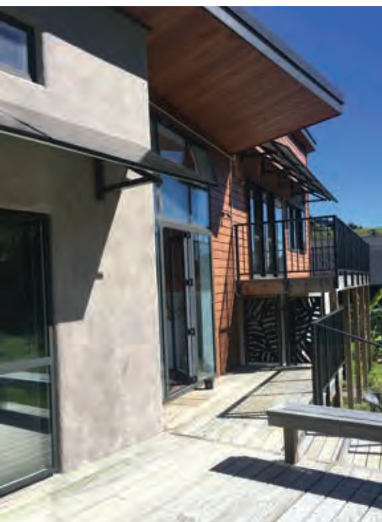
▲ Solar panels have a second use as shade for the windows in summer.
