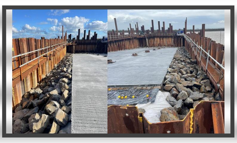
Once the rocks were all in place, we swept the boat ramp and blew out all the saw cuts with a compressor before applying Sika 11FC Sealant to all of the saw cuts.
