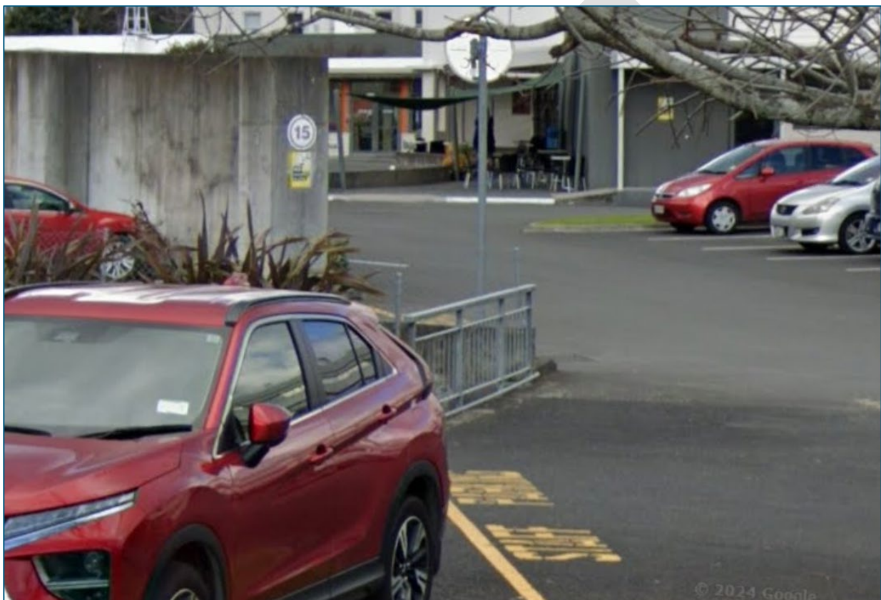
Figure 4-5: Concrete Walls on Karaka Stream (Taken from Google Streetview from Bella Street Looking East)
