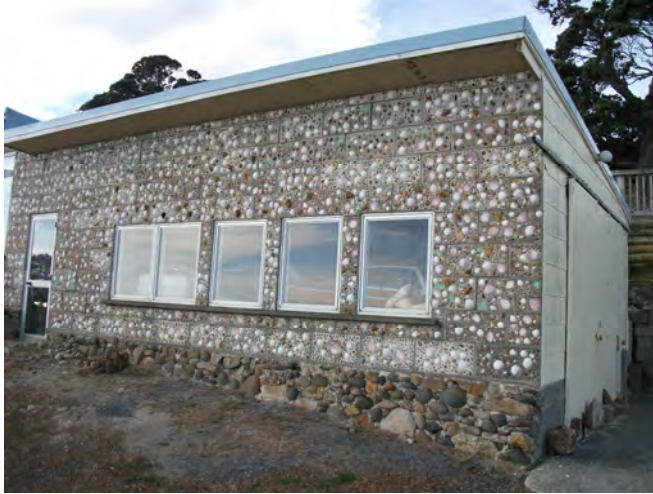
Western side - shell tile by door not set in correctly - shabby build of rock wall
