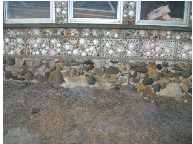
Western side - shell tile by door not set in correctly - shabby build of rock wall
