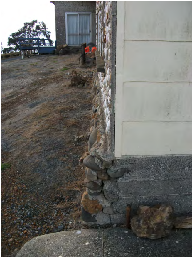
Shabby build quality of rock wall & concrete slab
