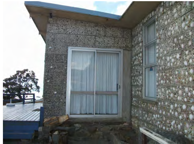
Wrong size Ali ranchslider - builder used plywood in corner
