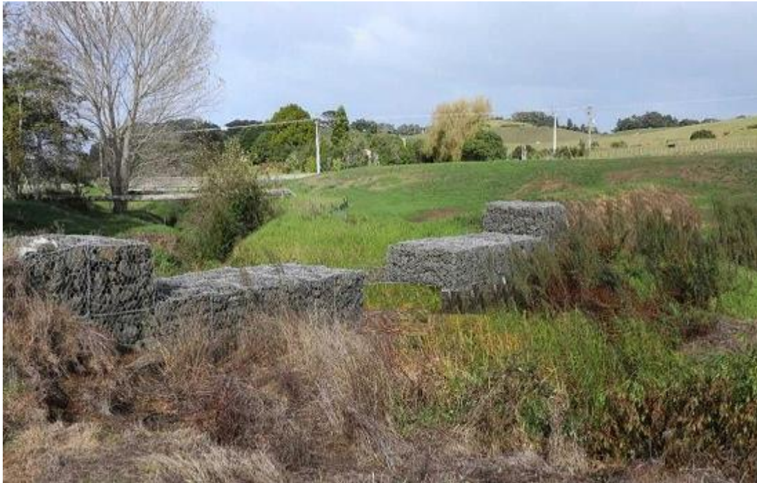
Figure 13 Gabion Weir Option
