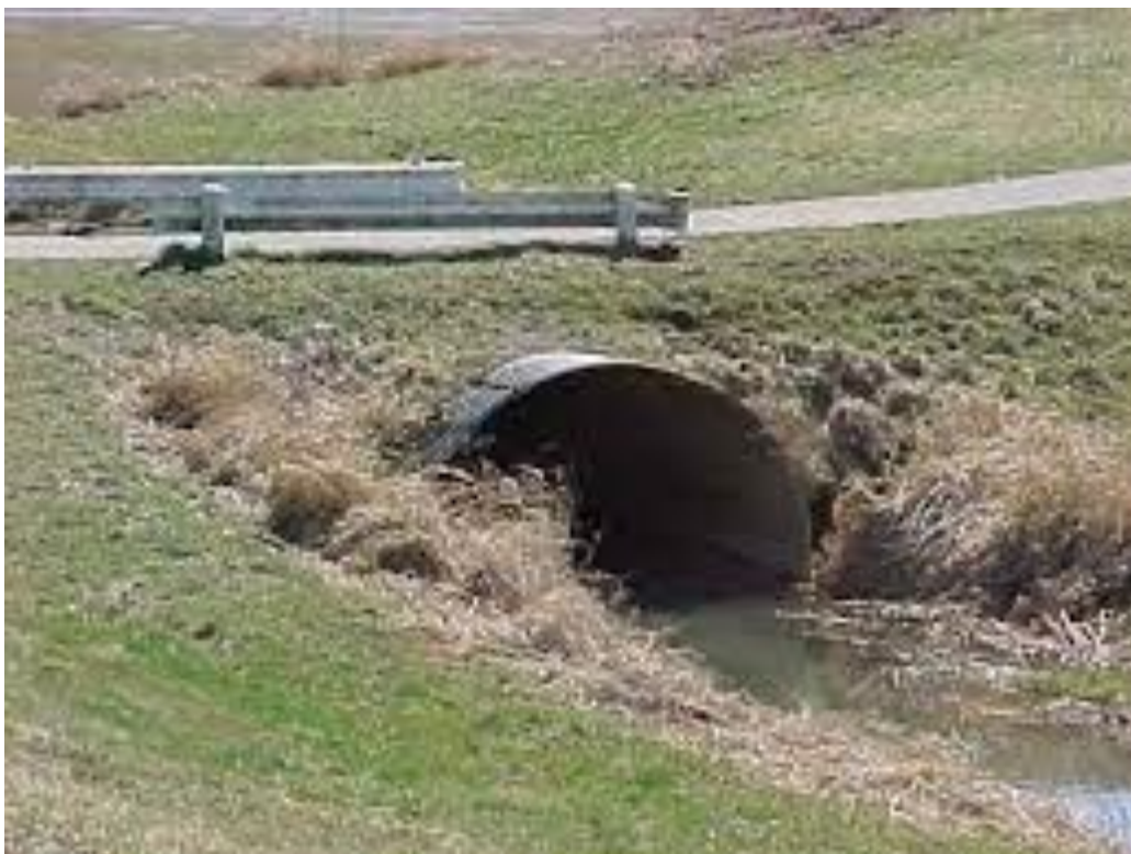
Figure 14 Culvert with Crossing Option
