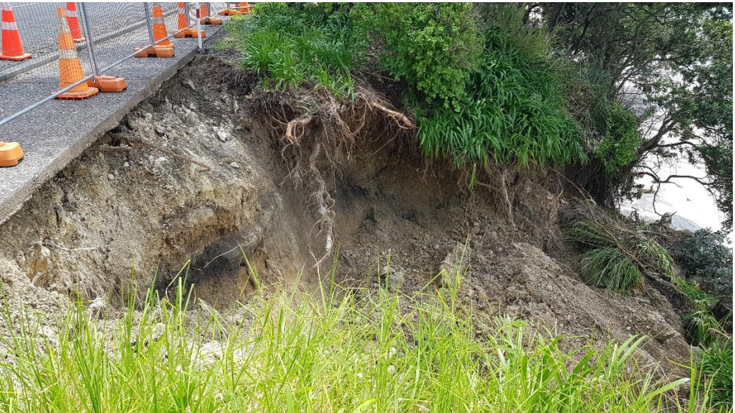
Figure 2: Looking up chainage at the scarp. Not the very outside edge of the concrete is undermined.
