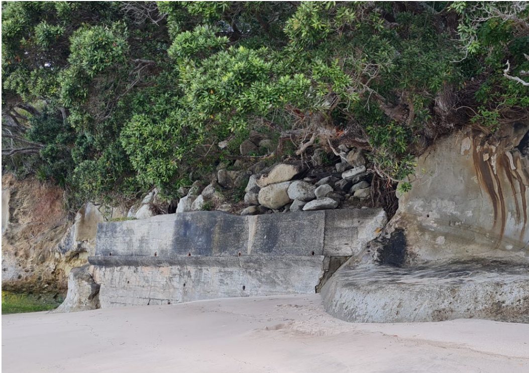
Figure 2-5. A concrete buttress protecting the cliff and road above it to the east of the slip.
