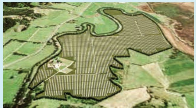
LODESTONE ENERGY'S PLANNED WHITIANGA SOLAR FARM.
