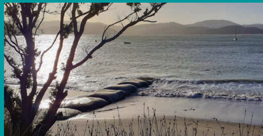
SHORELINE PROTECTION OPTIONS INCLUDE GROYNES, LIKE THIS ONE BEING TRIALLED AT FLAXMILL BAY, TO HELP MANAGE EROSION.
