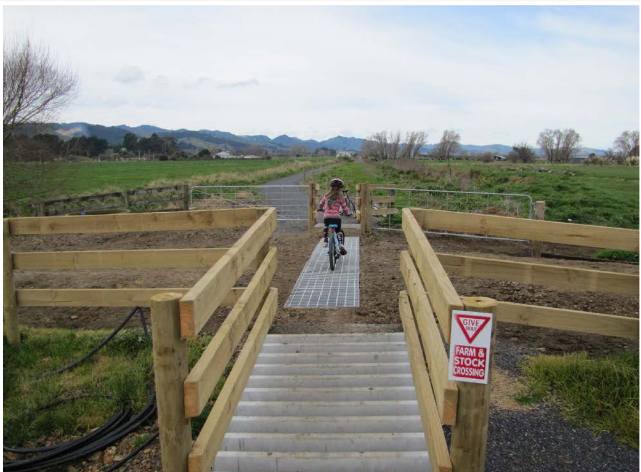
Hauraki Rail Trail - Matatoki area. Photo courtesy of Hauraki Rail Trail Trust
